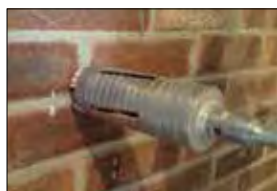
1. SELECT A 65MM CORE DRILL.
