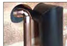
4. FIT THE ELBOW OVER THE COPPER PIPES.
