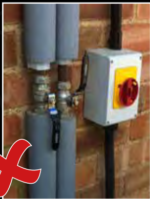
GREY/SILVER INSULATION FOR INTERNAL USE ONLY
