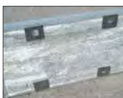
INSERT ALL 4 BASE PLATES THROUGH THE SLAB
