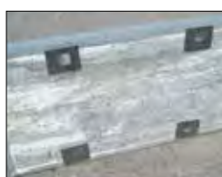
INSERT ALL 4 BASE PLATES THROUGH THE SLAB
