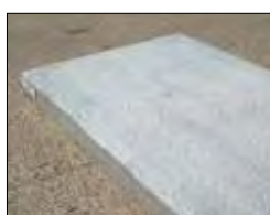
POSITION SLAB IN REQUIRED POSITION
